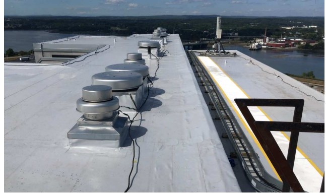
View of New Roof
