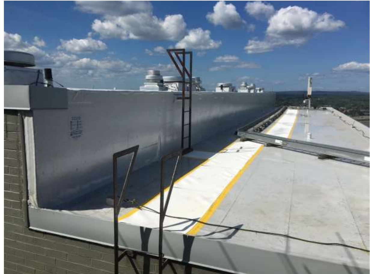
New Duro-Last Roofing Fully Adhered to Roof
