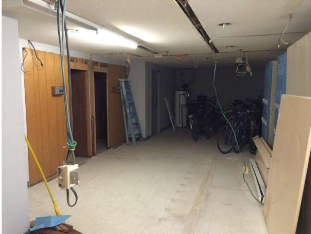
Old Locker Rooms/Saunas
