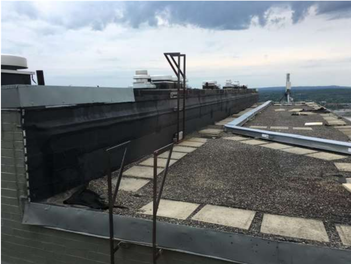
Old Rubber Roofing with Rocks and Pavers for Ballast
