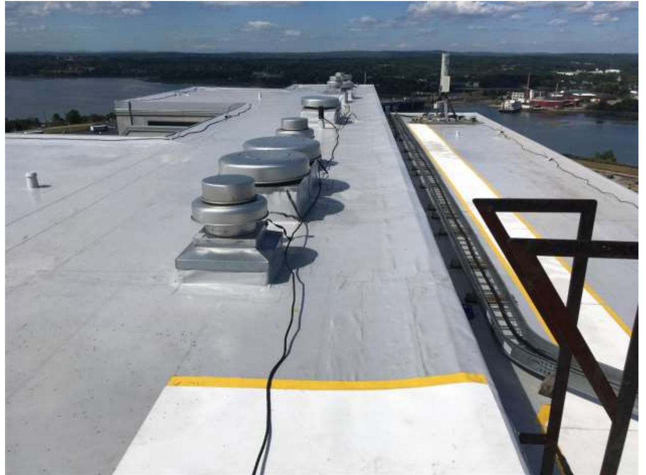
New Duro-Last Roofing Fully Adhered to Roof
