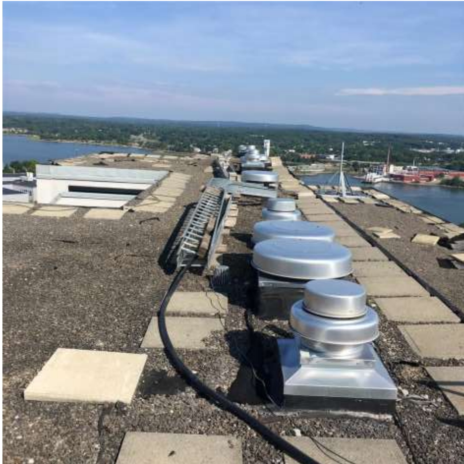
Old Rubber Roofing with Rocks and Pavers for Ballast
