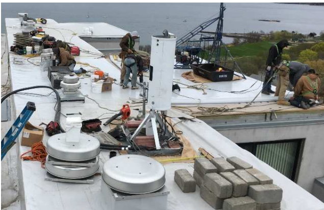
Completing Upper Section of Building 1
