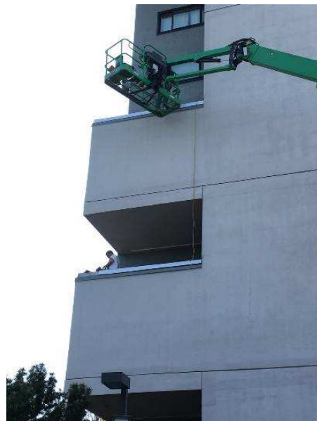
Building 1 Stairwell Roofs
