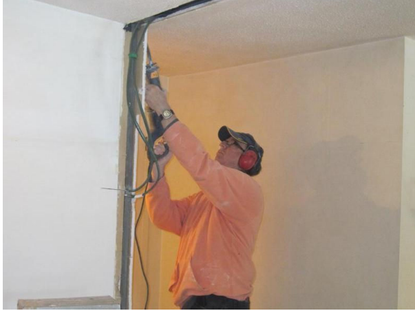
Demolition Phase for the New Fitness Room
